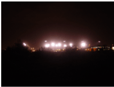
Sports facility NOT using full-cutoff luminaires
