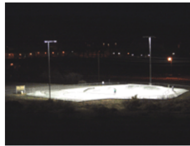
Sports facility USING full-cutoff luminaires
