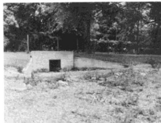
FIGURE 8 CRYSTAL LAKE DAM AND SPILLWAY
